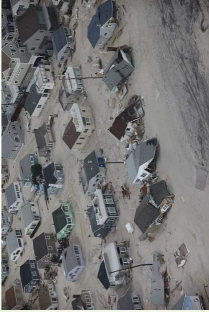
Aerial photo of damaged homes along New Jersey shore after Hurricane Sandy. Photo credit: Greg Thompson/USFWS. Public Domain
